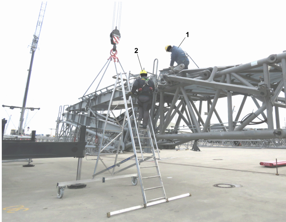
Fig.159590: Unpinning the N-assembly unit
