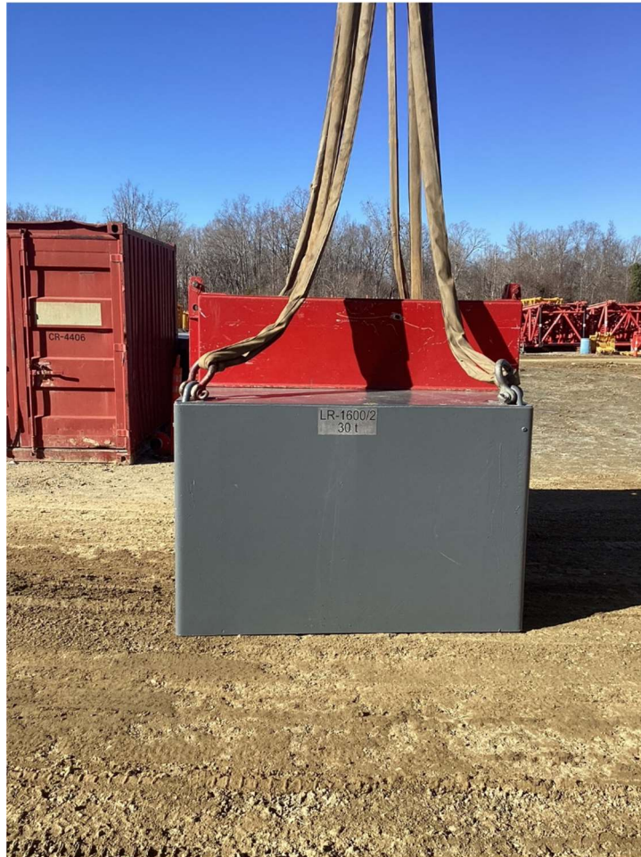
Picture 1 – Counterweight w/ Additional Ballast Weight Rigged in Test Configuration
