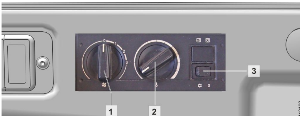
Control elements of heating
