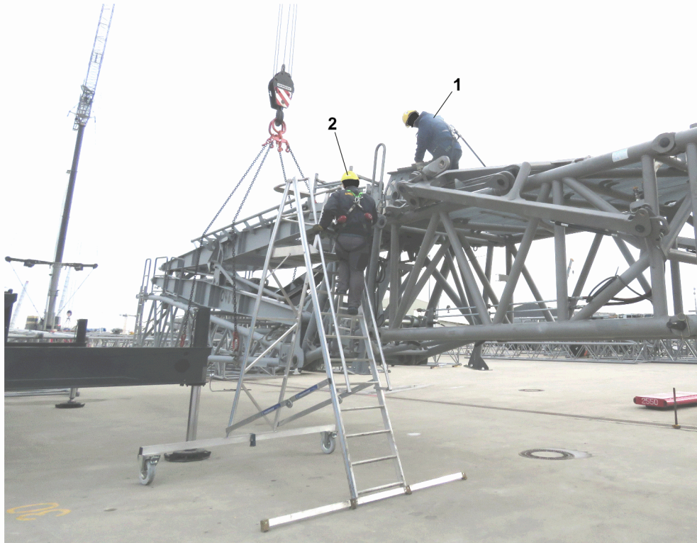
Fig.159590: Unpinning the N-assembly unit
