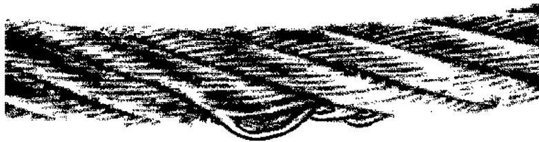
Fig.120991: Distorted or protruding strand
