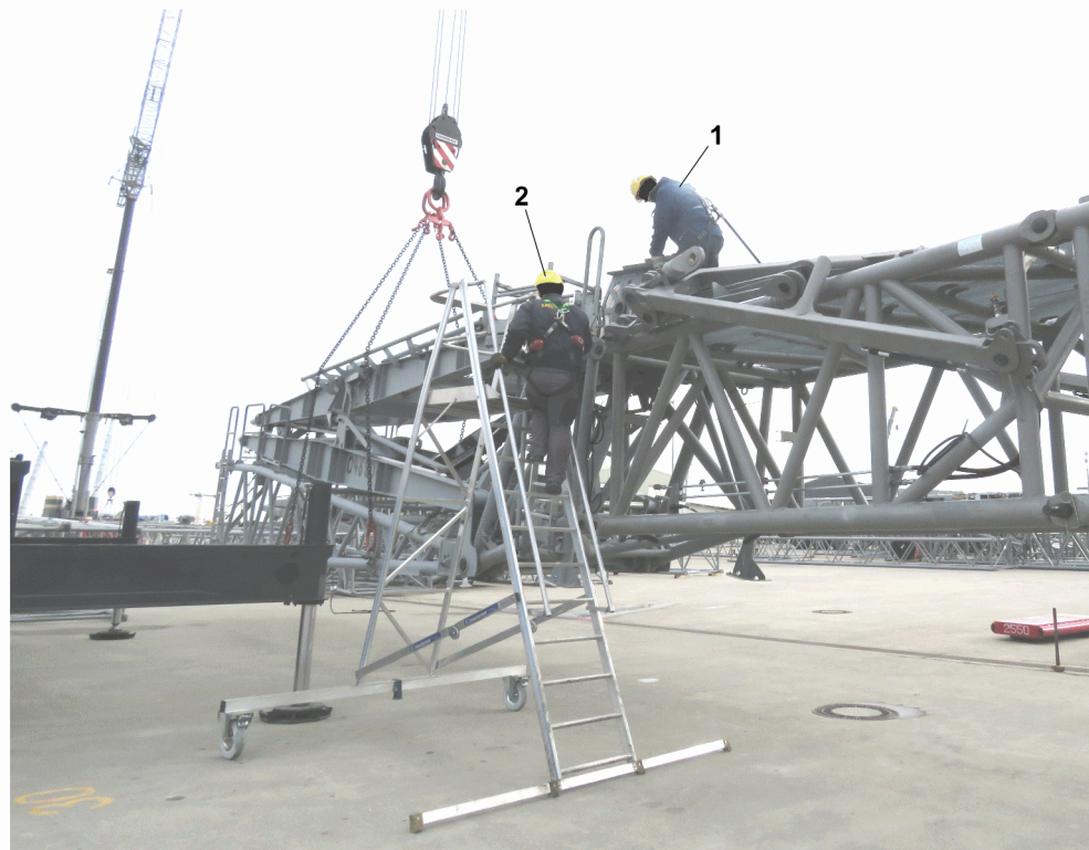
Fig.159590: Unpinning the N-assembly unit
